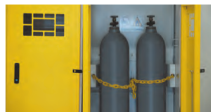
Plastic chain for fixing cylinders
