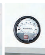
Differential pressure gauge
